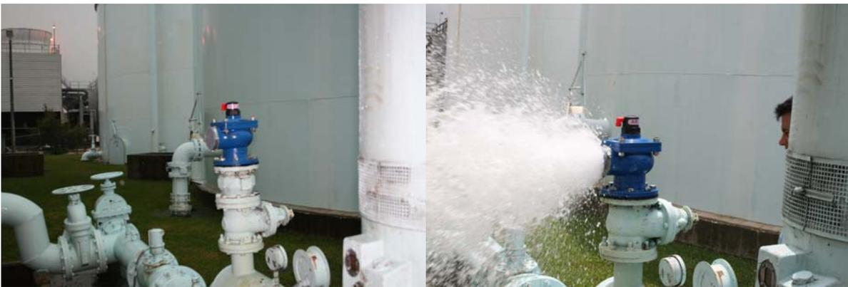
Pressure develops in the operating chamber, bringing about a controlled lowering of the sealing assembly, until the kinetic nozzle is completely closed. At this stage, the automatic small orifice air release valve continues to work, releasing air through its nozzle.
