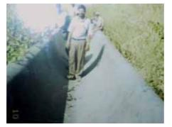
Figure 3: A steel pipeline, newly laid above ground (in India), collapsed when a drainage valve was opened for flushing, too fast.
